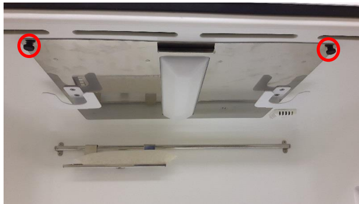
Figure 34: Ceiling Panel Thumb Screws
