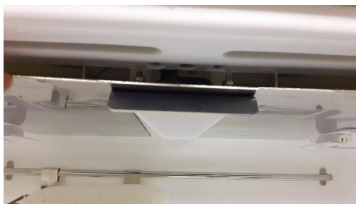
Figure 35: Ceiling Panel Handle and Grab Catch
