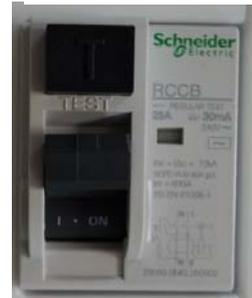
1. Workstation Residual Current Circuit Breaker (RCCB)
