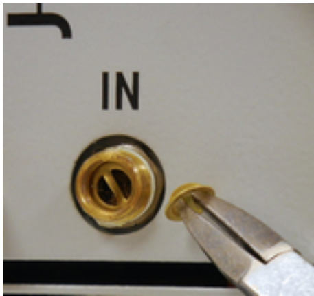
Fig. 68: Dirt trap installed, with pliers
