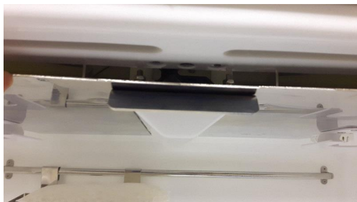
Figure 28: Ceiling Panel Handle and Grab Catch
