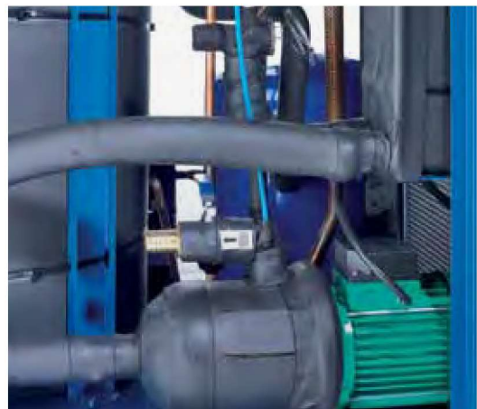
High-quality block pump for low-noise operation
