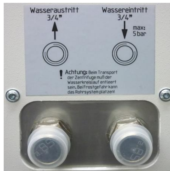
Fig. 8: Connections for the cooling water system
